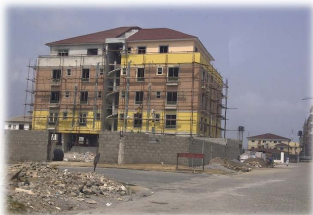
The above picture shows eight units of bedroom apartment flat at Oniru in Victoria Island Lagos. The building has been completed, and were designed and supervised by McGill Construction and Facility Management.
