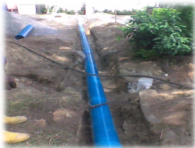
External works carried out at Eletu Ogabi in
