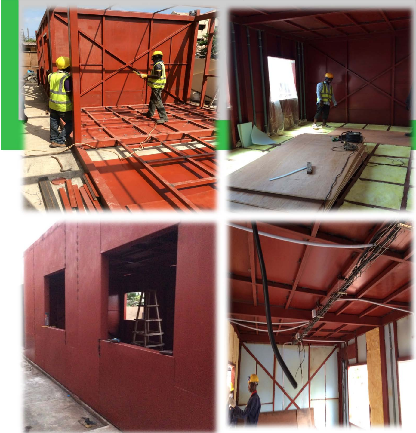
Self-drained Sound and Waterproof Portacabins at Construction Stage – Internal construction with Electrical Works and External Steel Walls - French School, V/I, Lagos
